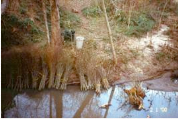
The left photo shows branch layers and pole plantings soaking in Branciforte Creek until installation with riprap (Santa Cruz County, CA). In the photo on the right, a triangular silt dike was used here to form a pond in a road ditch to soak live stakes (Sechelt, B.C.).
