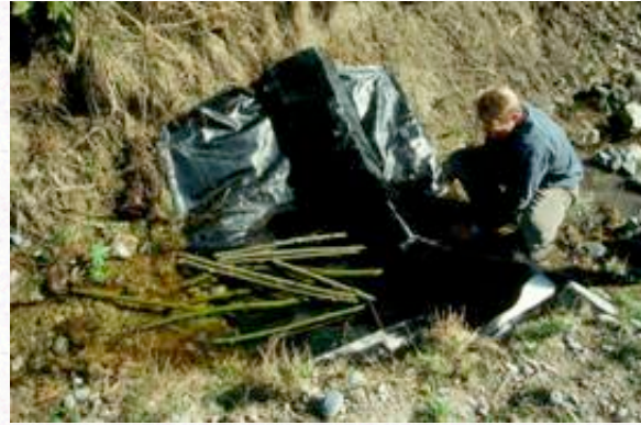
The left photo shows branch layers and pole plantings soaking in Branciforte Creek until installation with riprap (Santa Cruz County, CA). In the photo on the right, a triangular silt dike was used here to form a pond in a road ditch to soak live stakes (Sechelt, B.C.).
