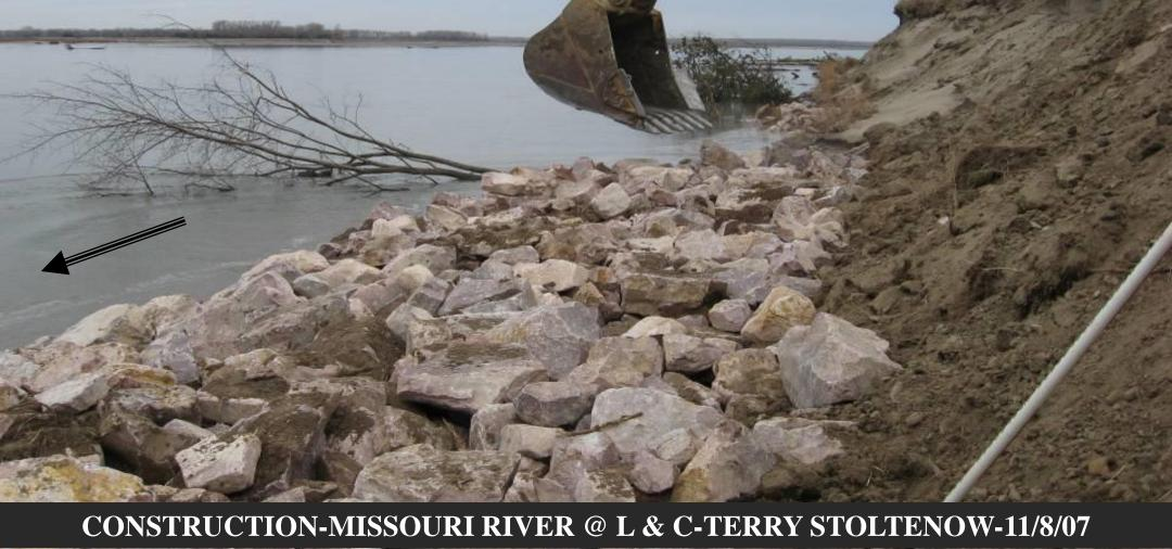
Looking US. Smoothing choke soil with the Bobcat. Minimum of 6 inches of soil choke, but contractor applied 12 inches almost everywhere. Some settling will occur.
