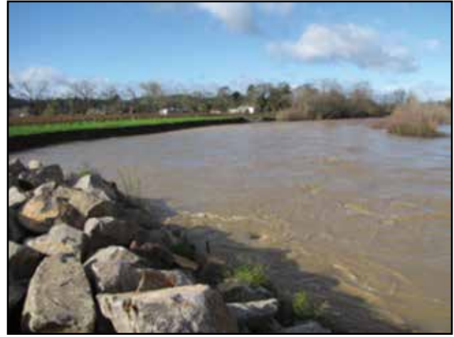
The site has experienced several floods. This flood is in March 2011.
