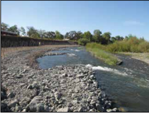
Above: Project completed on October 11, 2010. Here terrace has pole plantings (willow and cottonwood) installed and counted. Note the poles are over 9-ft tall.
