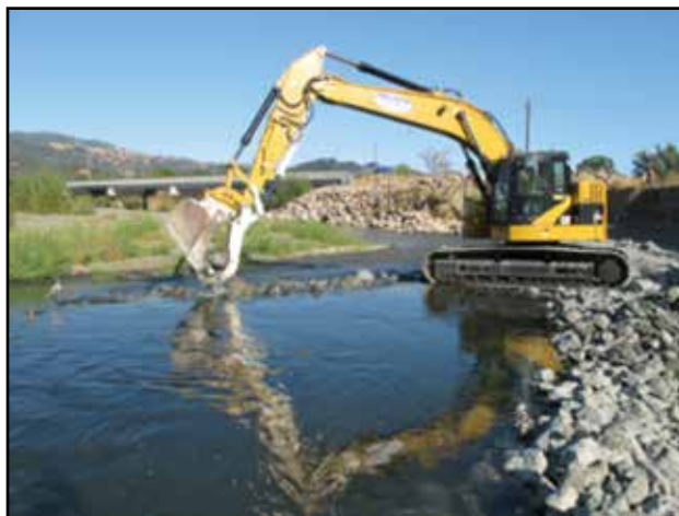
Clean self-launching rock, installed by skilled operators assured no turbidity issues.
