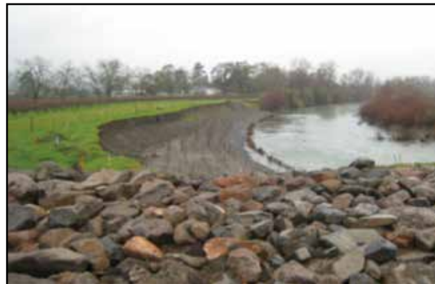
After 15 days the flood receded and no erosion had occurred.
