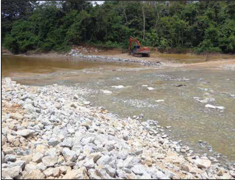
Downstream section completed. Note that the eroded and scoured right bank did not need protection - it became a flood terrace that refilled and maintained itself.
