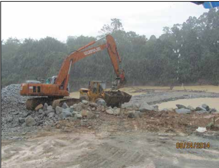
Above: Very hot and humid, followed by 1"/hr rainstorms. In the background - turbidity of the river went from 18 NTUs to over 1800 NTUs in 3 hours. Below: We placed 6000T of rock. Here the crew is working through a heavy rainstorm.
