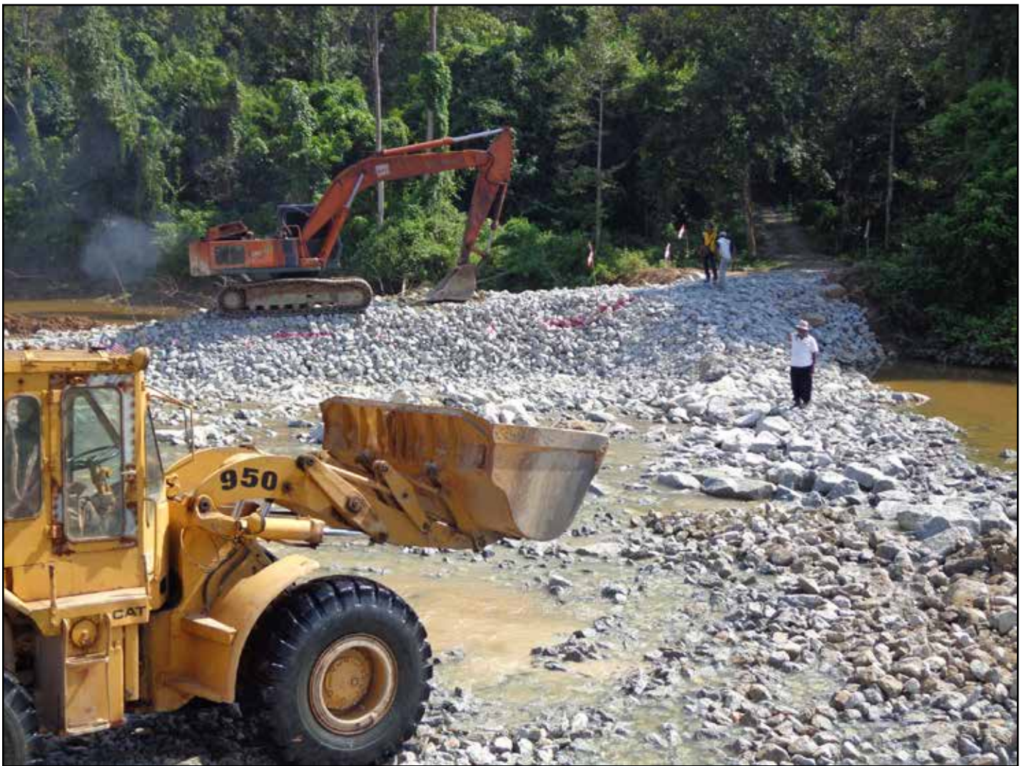
The weir crest nearly complete, about 18" to go.
