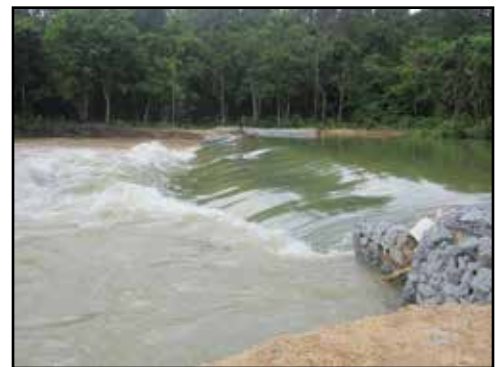
Gabions with water over.
