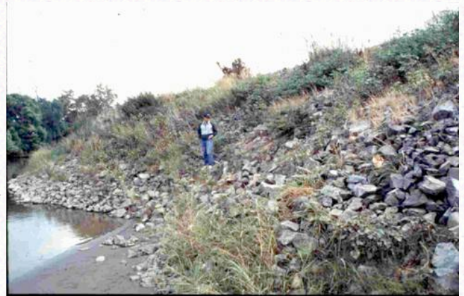
Figure 1. Riprap Revetment, Sacramento River, California. A form of resistive bank protection.
