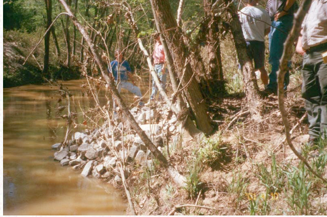
LPSTP (under people) with Stone Deflector (spur) after several years.
