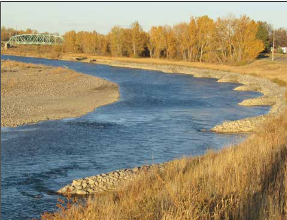
Above: Rock Vanes on Old Man River, 3 years after installation. No damage from record storm. Below: Old Man River, Fort Macleod, AB. Seven months after construction, the Rock Vanes and Flood Terrace experience a 30-yr flood. The high erosive energy and thalweg is directed streamward off the ends of the vanes.
