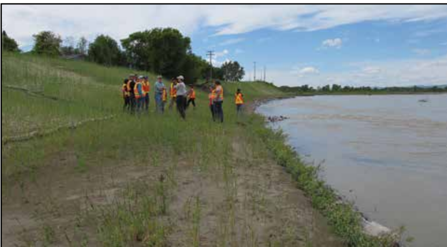
Above: Rock Vanes on Old Man River, 3 years after installation. No damage from record storm. Below: Old Man River, Fort Macleod, AB. Seven months after construction, the Rock Vanes and Flood Terrace experience a 30-yr flood. The high erosive energy and thalweg is directed streamward off the ends of the vanes.
