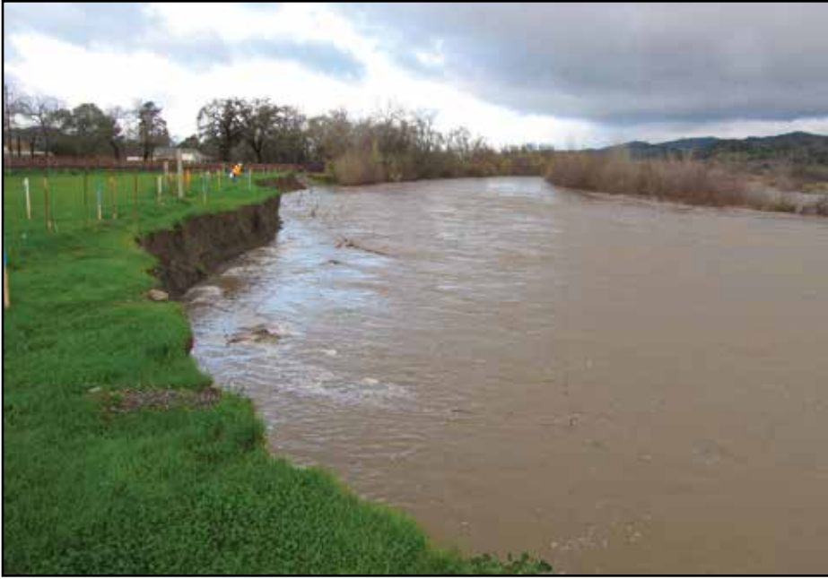
On December 29, 2010, 2 months after completion the Russian River at Geyserville Bridge gets high flows (>10,000 cfs), 9 ft. over the Rock Vanes.
