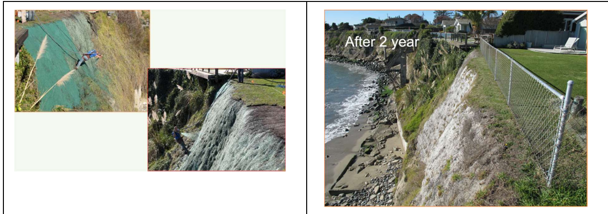
Figure 1 John's brothers house on Opal Cliffs Drive in Santa Cruz, CA needed innovative steep slope soil stabilization. Here John applies Green Armor System to the 'cliff'. The stabilization methods stopped erosion for over 4-yrs, until the property was repossessed. The native maritime blend establishment was sparse, probably for failing to do soil test.
