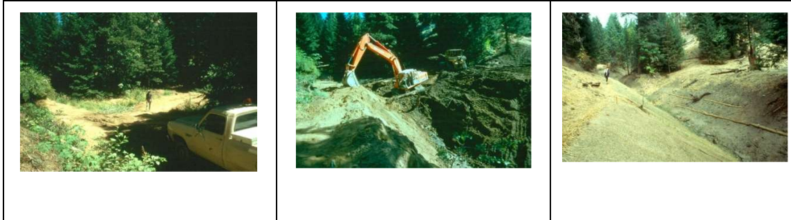
Figure 2 This potential gully site treated with landform grading - logging road removal involved removal of "dozer placed DG sediment from the waterways. This was one of our first examples of the dozer - excavator team "restoring its way out of the watershed.
