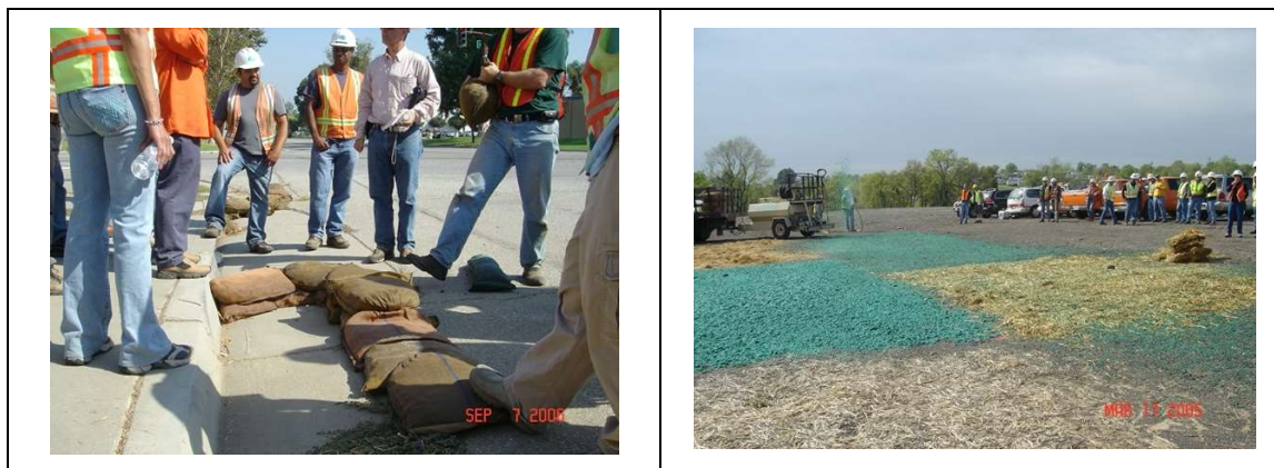
Figure 3 John, David Franklin, and Colin Ewert demonstrate to CT staff the proper gravel bag barrier placement, so not to plug curb inlet and demonstrating the use and application rates of hydromulches and straw mulch.
